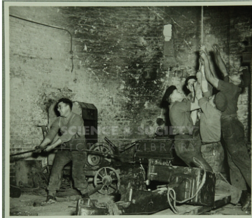
Inside the Shot Tower. Men of the 245 Armament Battery RA pulling down the steel-rope with which to hoist to the top parts of the AA Gun mounting for the umbrella shaped aerial of the radio-telescope
